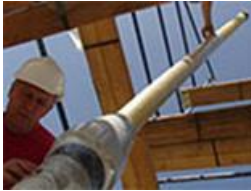
Final Preparation before Insulator Fixing
