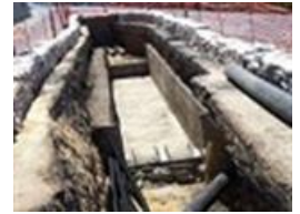
End of Cable Pulling
