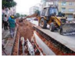
Backfilling
