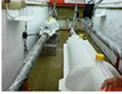
Complete Joint with Coffin Box
