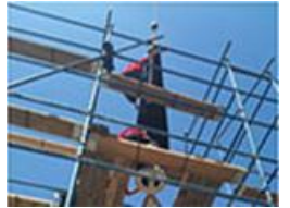
Insertion of Insulator
