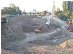
Excavation of Trenches
