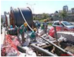
Start of Cable Laying
