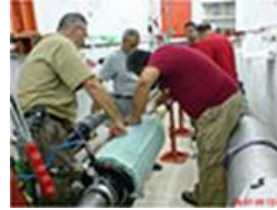
Pulling Cable into Joint Bay
